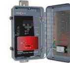
8 kV Capacitor Bank w/ M6280 Controller
