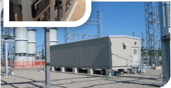
New Protection, Control & Telecom Building
